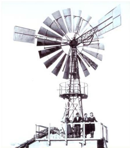
Fig. 1 - Wind engine built in Capracotta in the early 20th century to run a disk saw and an alternating saw (Photo dated 1936)
